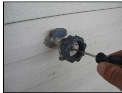
Figure B-2: Turn the water off inside the house at the main shut-off. Then remove the screw that retains the faucet handle and pull the handle off.
