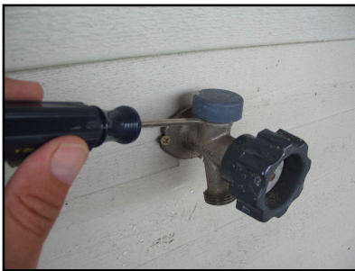
Figure A-1: Using a flat bladed screw driver pry against the metal ring formed on the faucet body and push the plastic dust cover cap upward. This will expose the anti-siphon valve.
